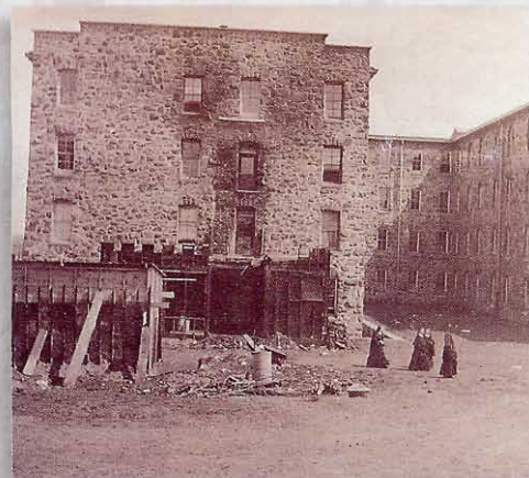
Sisters view the aftermath of the 1913 fire in the boiler room/science laboratory building.
